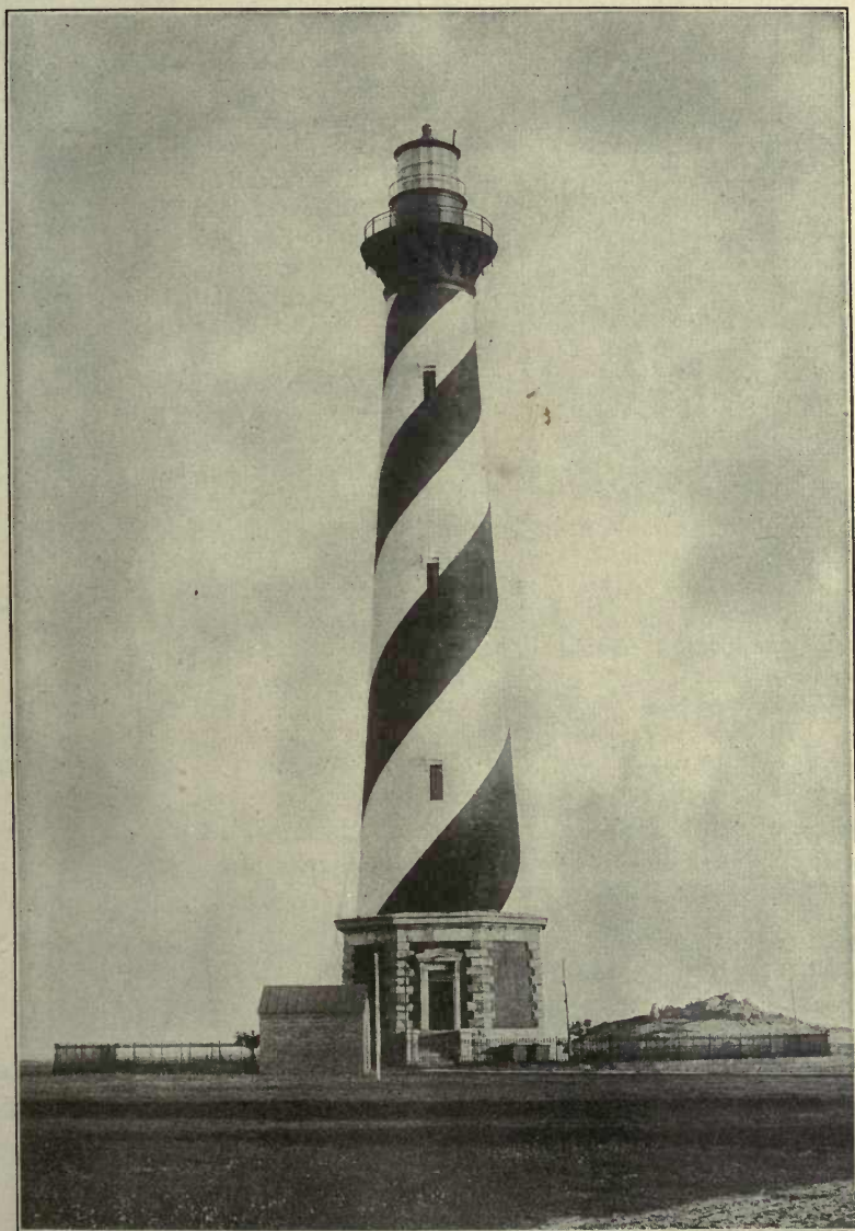
Cape Hatteras Light Station, N. C.
